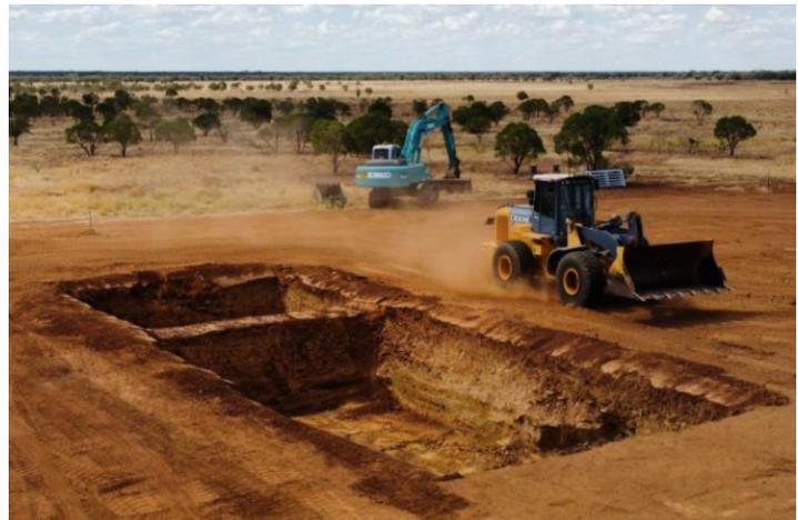
Figure 2 – drilling lease construction
